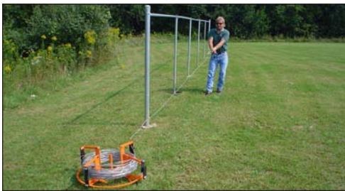
The Hog Stringer dispenses bottom tension wire with ease, while the Hog Hangers slide easily on the top rail to temporarily hold the fence.
